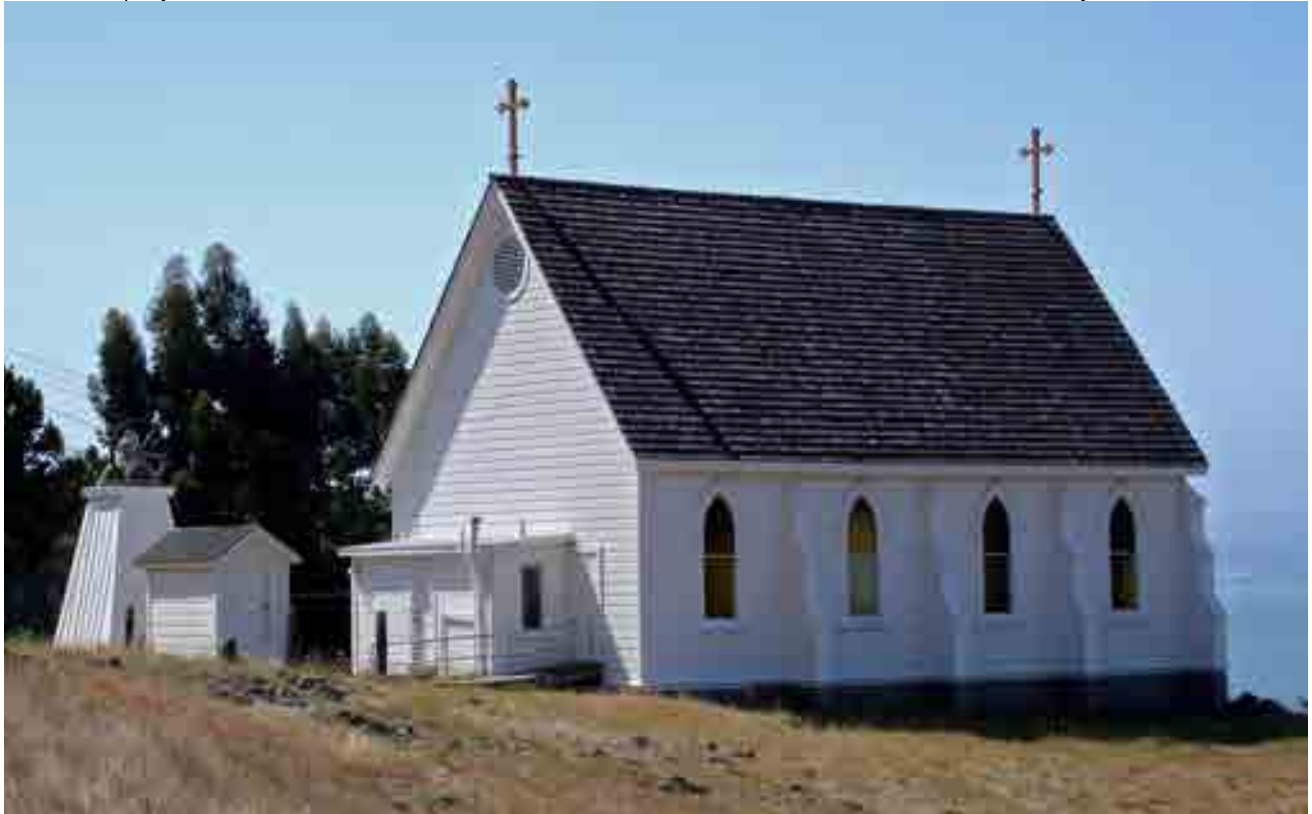
Figure 6. North-east view showing roof details as well as the sacristy attached to the rear of the building, handicapped compliant ramp, outhouse before conversion into a restroom and bell tower now painted to match the rest of the buildings, May 2007.
