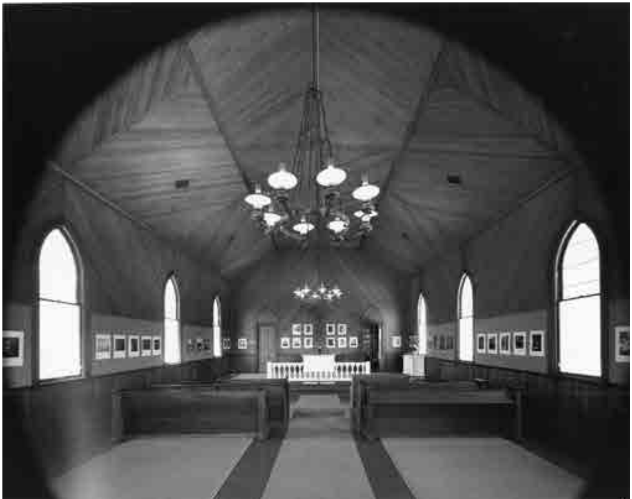
Figure 7. Interior view in 1975 showing redwood tongue and groove paneling set at oblique diagonals to create a herringbone pattern, reproduction chandeliers (1966), east entrance doors and other interior details.
