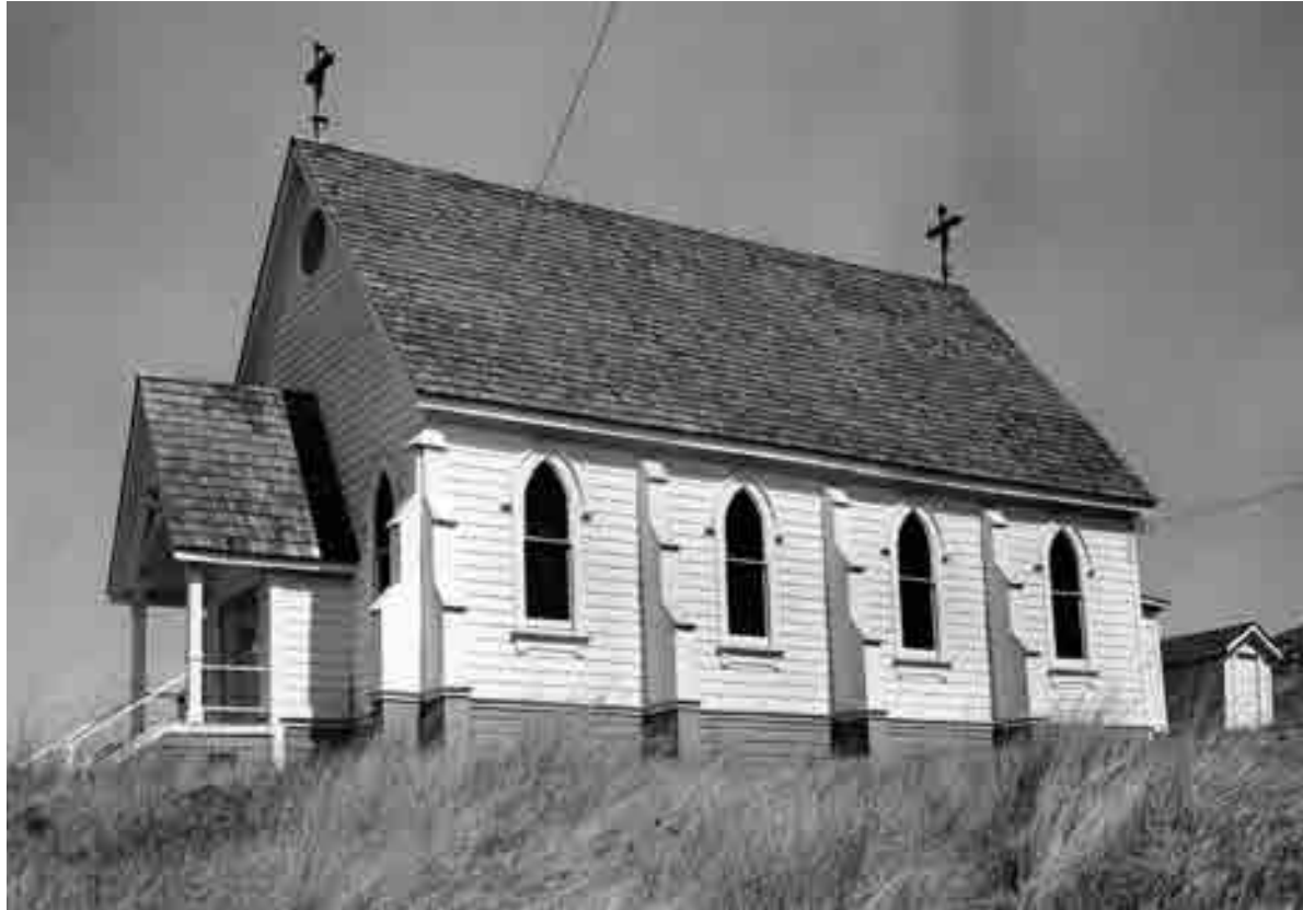
Figure 5. South side view showing roof, buttresses and window details, 1970.
