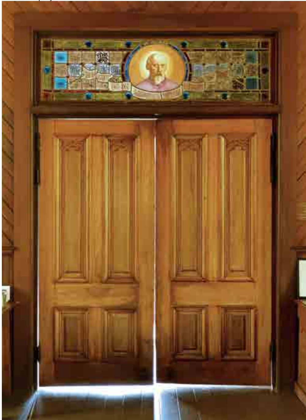
Figure 9. Interior photo from 2019 showing the double swinging, four-panel, mortise and tenon Douglas fir doors which separate the nave from the narthex are set beneath a stained glass panel featuring the likeness of St. Hilaire.
